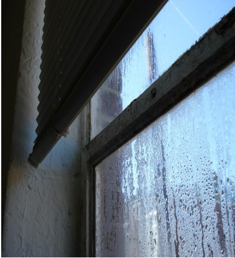
Condensation on cold window
